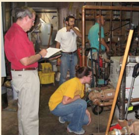
A Green Building energy audit at Northwood Christian Church, Indianapolis.
