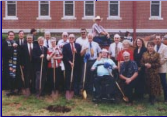
Members of Kingman Christian Church, Kingman, Kansas, break ground on their new addition. The facility will allow older members and those with disabilities better accessibility throughout the building.
