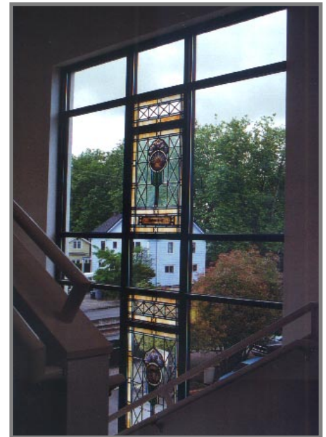
Stained glass windows that would have been concealed by new construction were relocated to the new stairway/elevator addition.
